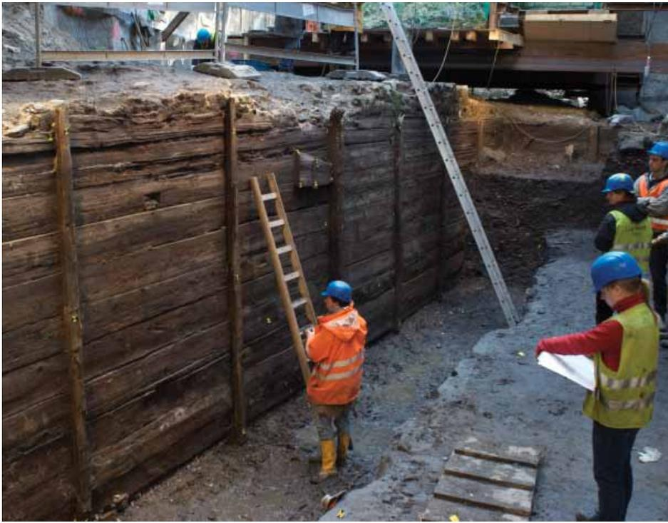
**ABOVE** The wooden shuttering on the inner-face of the Roman town wall's foundation was extremely well preserved, thanks to the water-logged conditions of the soil at near ground water levels.
